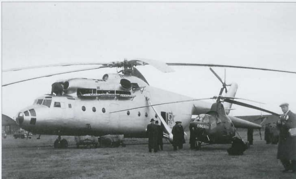
Above: The Mi-6 prototype dwarfs its stablemate, a Mi-1TU trainer, at Zakharkovo airfield. Note the open cowlings serving as work platforms and the windowless forward entry door.
