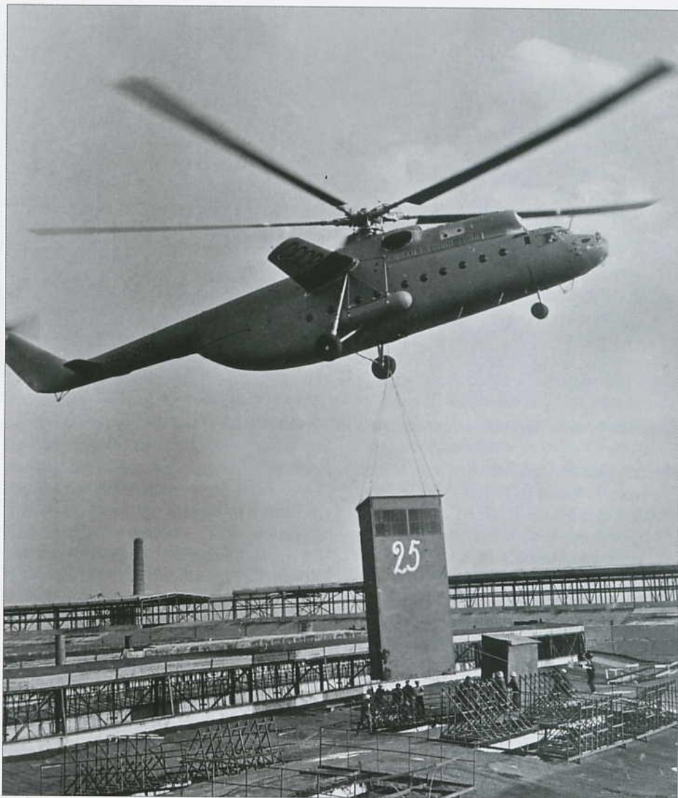
Above: The Mi-6 was often used as a 'flying crane', as exemplified by CCCP-21192 (c/n 9684205V) of the Komi CAD installing a ventilation outlet at an industrial construction site in 1969.
