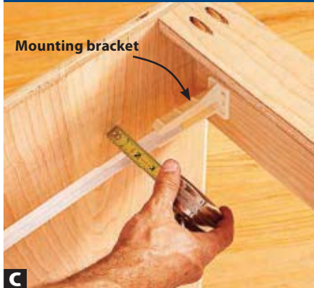
A Hold the slide perpendicular to the face frame—we like Kreg's magnetic mounting tool, shown—while attaching with screws.
