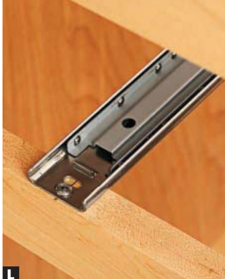
L Mount the slide \frac{1}{32} " back from the front of the face frame. You might need to angle the screw slightly to avoid the frame above.
