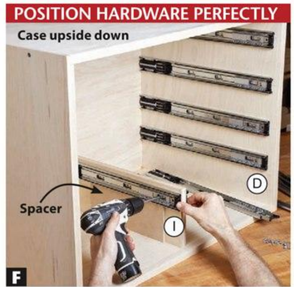
F Work from the highest to lowest slides. When reaching the lowest slides, remember to add the mates to each side of the divider (I).
