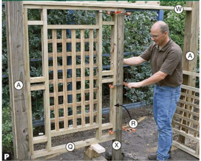
P Clamp the screen post (X) to the upright (R). Screw the upright to the post, then screw the remaining screen (Q-V) in place.
