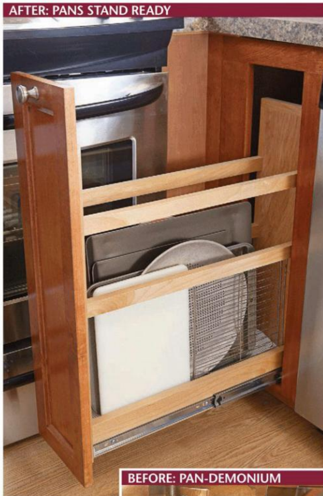
Position the rails to support your flat pans, cookie sheets, and cutting boards. The bottom rails act as the sides of a long tray.
