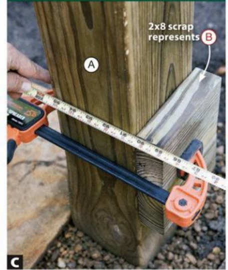
C Clamp a 2 × 8 scrap to each post to represent the inside beams (B) when measuring for the length of the crossbeams (C).
