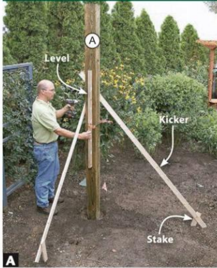
A Brace the post (A) with kickers and stakes. Check for plumb in both directions before and after adding concrete to the hole.
