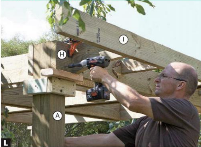
L Position the end of the outside beam (H) flush with the outside face of the post (A). Drill pilot holes and drive lag screws.
