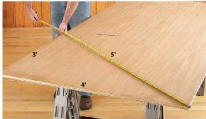
If the diagonal measures 5' at the 3' mark of a 4' wide sheet of plywood, then the corner is square. Just remember: Not all plywood is exactly 4' wide.
