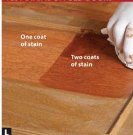
L First test stripper on the varnish. Then see how different stains and multiple stain coats will look on the face frames.
