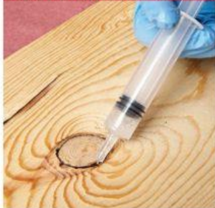
Small gaps in loosening knots may require injecting epoxy with a glue syringe in order to lock in knots.
