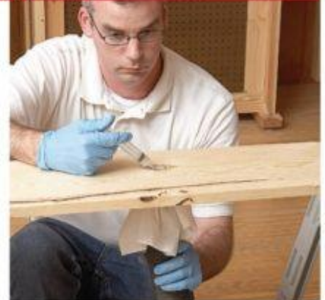
To draw the epoxy into the gaps, use a shop vacuum. Protect the hose by rubber-banding a paper towel over the end.
