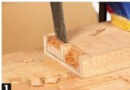
1 Remove the socket waste with a bench chisel, keeping \frac{1}{16} " from the scribed sides and back.
