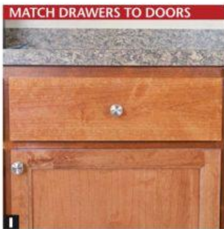
I By installing the cabinet doors first, you can align overlay drawer fronts with doors of the same width.
