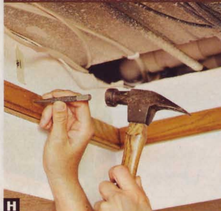
NAIL WALL STRIPS IN PLACE
