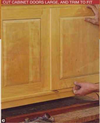
The hutch doors were purposely cut larger than the opening. Trimming down the doors takes time, but it's easier and quicker than correcting a gap during installation.
