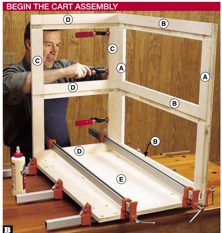
B Glue and clamp a side frame (A/B), end frame (C/D), and the bottom shelf (E) together, making sure you close the frame corner joint by drawing the end frame tightly in the rabbet in the side frame.
