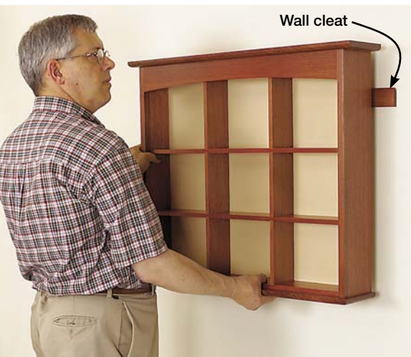
A wall-mounted cleat provides a wide, stable surface for mounting this display shelf. The wall cleat visible to the right will be hidden by the shelf.
