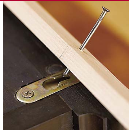
For perfect spacing, make certain the tips of the nails are centered within the narrow part of the keyhole.
