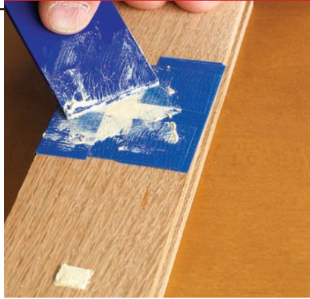
Press putty into the damaged area enclosed by two layers of masking tape, which also keeps excess putty off surrounding wood.
