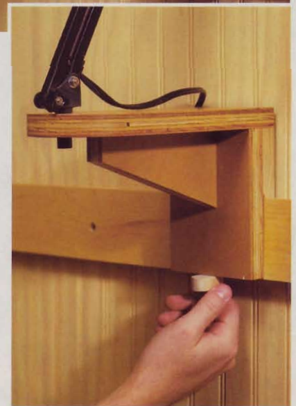
Rotate the turn button to secure the light support to the wall cleat.
