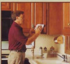
Cabinet Refurbishing - cleaning, degreasing, repairing and polishing
