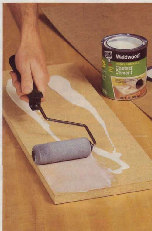
Spread water-based contact cement evenly on your substrate. When the adhesive becomes tacky, apply the plastic laminate, and then press it down firmly with clamps and cauls.
