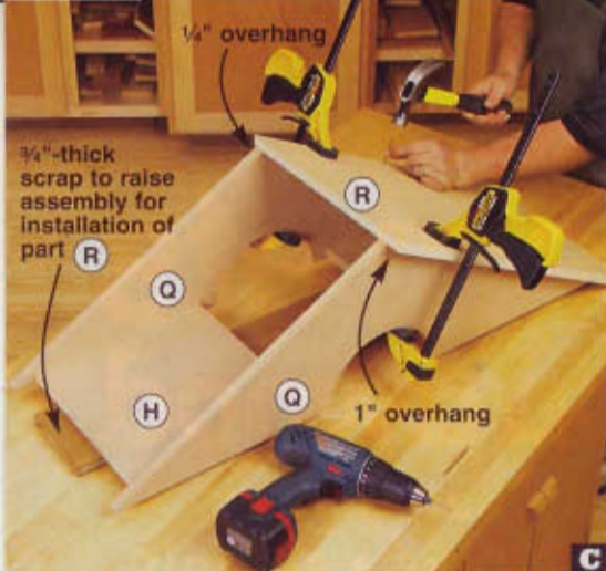
With the roof panels (R) positioned so they overhang the roof supports (Q) 1" in the front and 1/4" at the back, drill pilot holes, and nail the panels to the supports.
