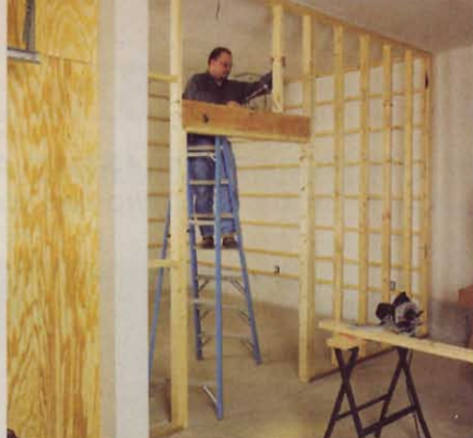
We walled off one 15x22' bay from the rest of the garage to create shop space, and then covered the drywall with a more durable, attractive surface: beadboard pine plywood.
