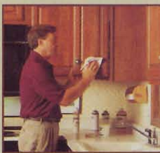
Cabinet Refurbishing - cleaning, degreasing, repairing and polishing
