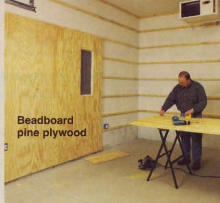
We walled off one 15x22' bay from the rest of the garage to create shop space, and then covered the drywall with a more durable, attractive surface: beadboard pine plywood.
