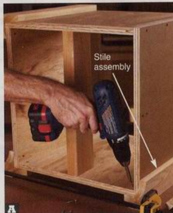
A With the stile assemblies clamped to the box (no glue), drill countersunk shank holes in the box, and drive the screws.
