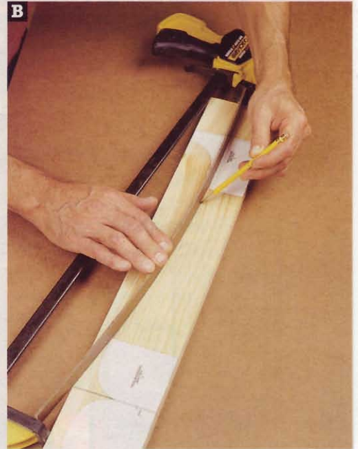
Bend a thin strip of wood to form a shallow arc, and draw curved lines connecting the end and center patterns.
