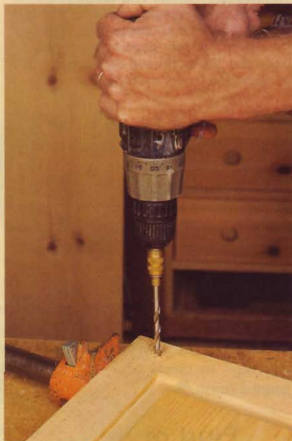
Once the joint is glued and clamped, Bill drills a \frac{1}{4} " hole that travels through the mortise-and-tenon door frame. Use a block of scrap on the underside to prevent chip-out.
