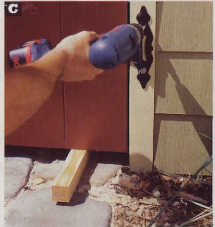
First, mount the hinge's strap on the gate. Then, using the holes in the hinge's T as guides, drill pilot holes in the surround and drive in the lag screws.
