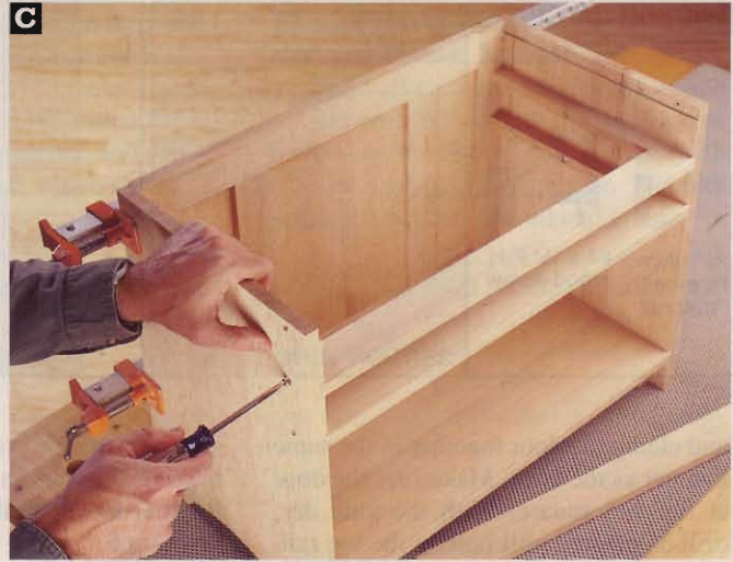
With the back panel glued and clamped between the sides and the bottom screwed in place, drill pilot holes, and drive in the screws that fasten the rails.
