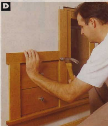
Position all vertical and horizontal trim to leave a 1/4" reveal around the boxes.
