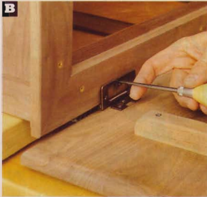
To locate the hinge positions on the back top trim (N), set the chest on 1½"-high support blocks (we used 2x4s). Position the top (P) as shown.
