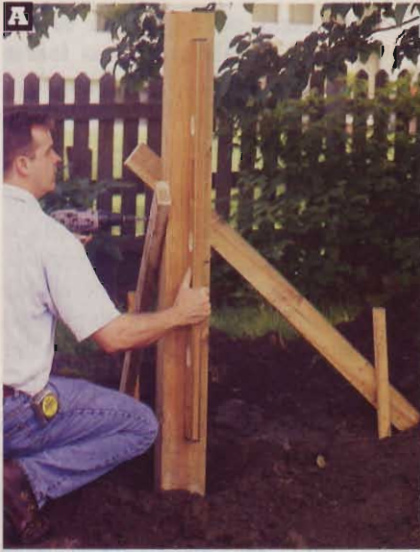
Check the post on adjacent sides for plumb. Fasten 2x4 braces to the stakes and the post with screws.
