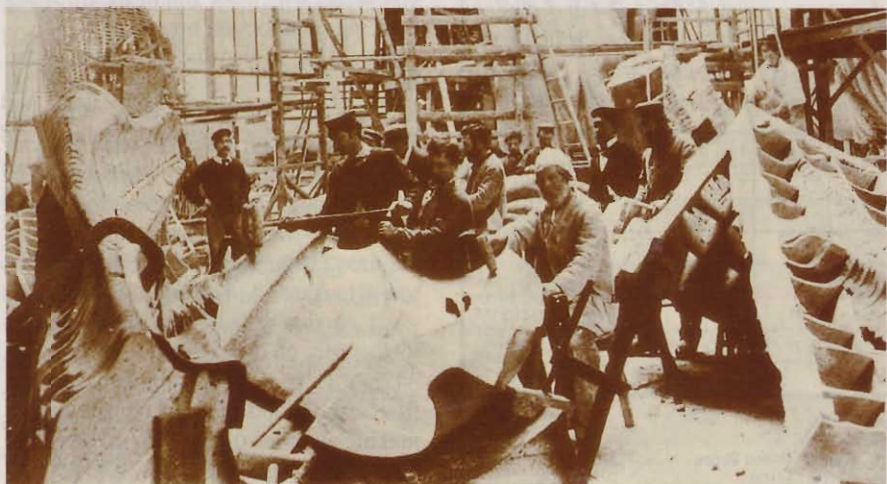
Some 310 huge sheets of copper were hammered into shape against intricate wooden molds to shape the skin of the Statue of Liberty.
