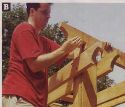
Drop the cross joists in place over the main joists.
