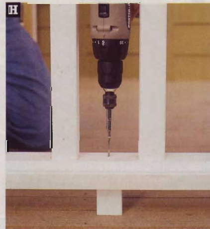
To prevent sagging install 4"-long pieces of baluster stock between the deck and bottom rail assembly.
