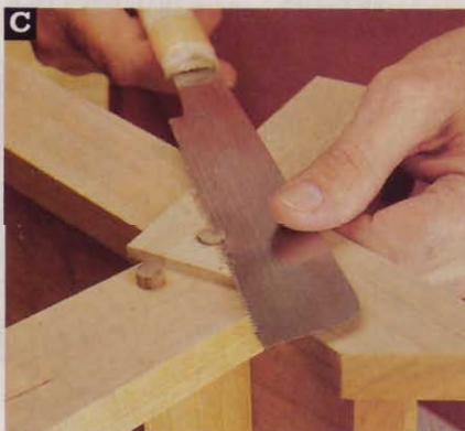
Drill a \frac{3}{8} " hole in the end of a \frac{3}{16} "x2x6" board. Place the board over the protruding plug and saw and sand it flush.
