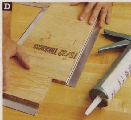
Align the plywood top and sheet metal, then place weights on the top. Let the silicone cure before bending the metal.
