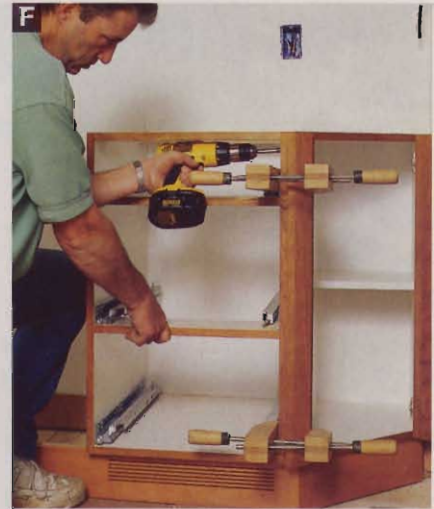
F If you build your base cabinets carefully, and set the toekicks perfectly level, this step is easy. Clamp adjoining units together, and attach them with screws.
