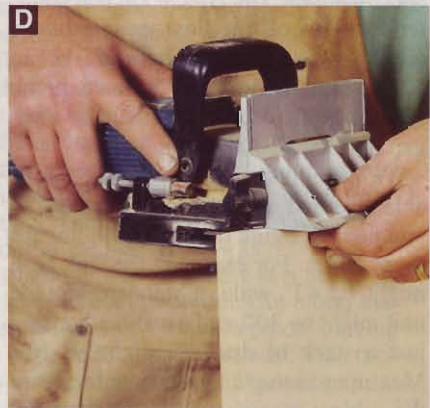
D Keep joinery simple and avoid measurements completely, when possible. Here, the biscuit joiner is lined up with the edge of the cabinet side.
