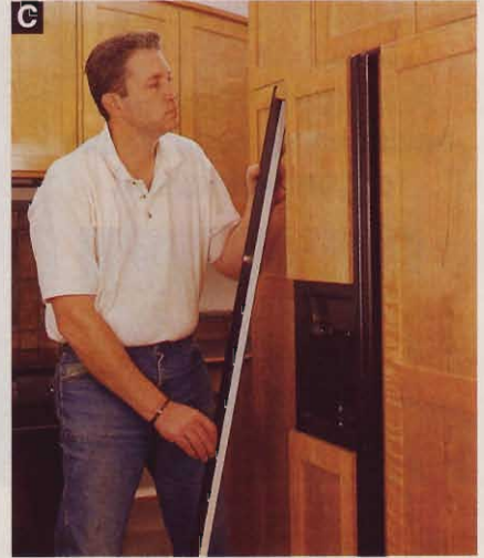
C Attach the trim kit's flange to the outside edges of the doors (double-faced tape holds them securely).
