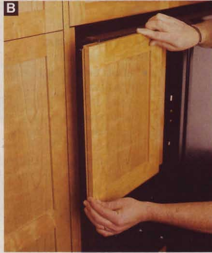
B Then, slide in the panel, being careful to insert the refrigerator's panel-retaining lips in the panel's groove.
