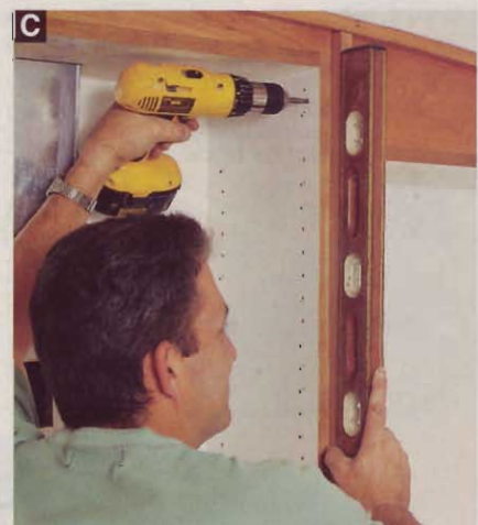
C There's no need to clutter up the inside of a cabinet with lots of screwheads. Fasten adjacent cabinets with screws placed inside hinge or shelf holes.
