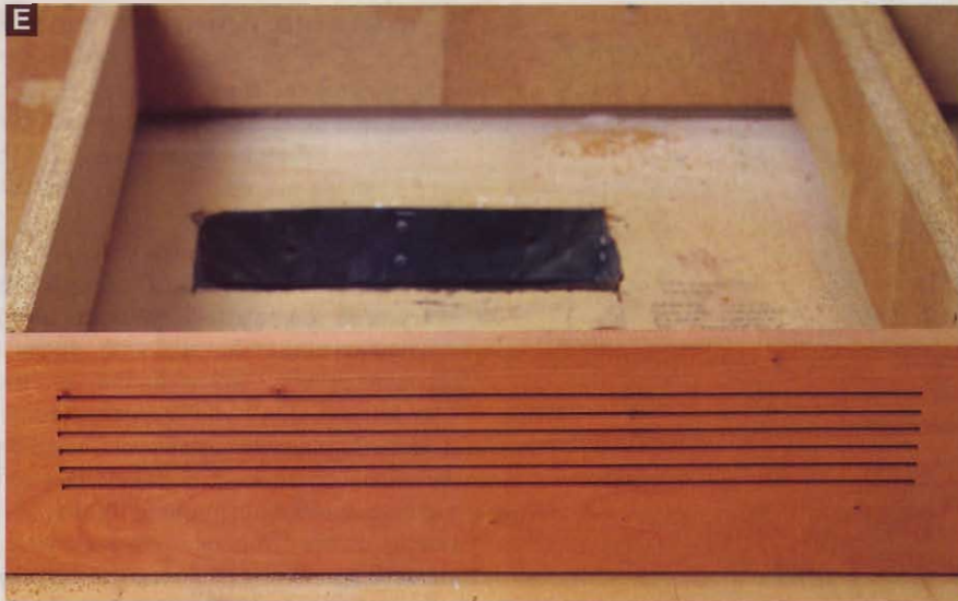
E Simple saw kerfs produce a clean-looking heating-and-cooling register. Seal the gap around the inside of the compartment with caulk.
