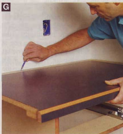
Scribing with a pencil transfers wall irregularities directly to masking tape on the countertop.
