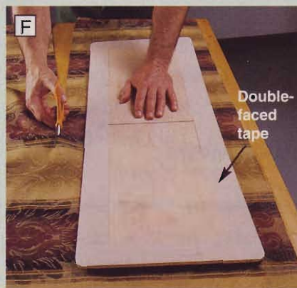
F Align the back panel on the fabric, and trim the fabric so it wraps the panel edges and covers the double-faced tape.
