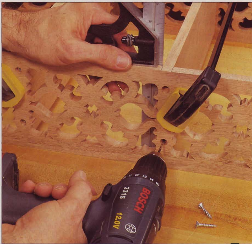
Align the shelves with a square, clamp them in place, and drill the \frac{7}{64} " pilot holes using the shank holes as guides.
