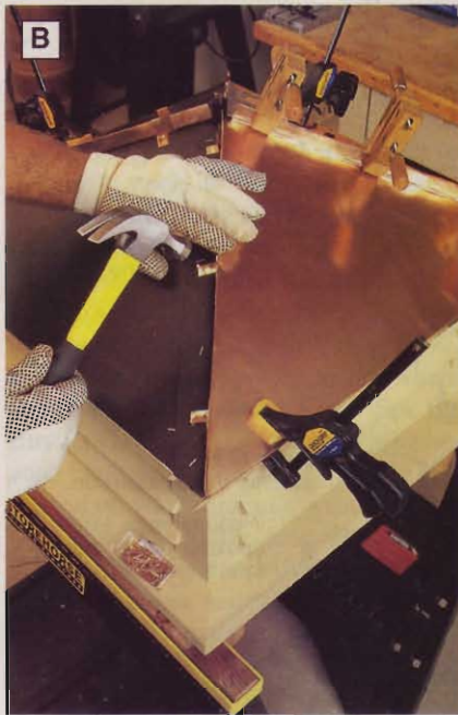
B Use the copper clips to secure the copper roof panels to the roof sheathing.
