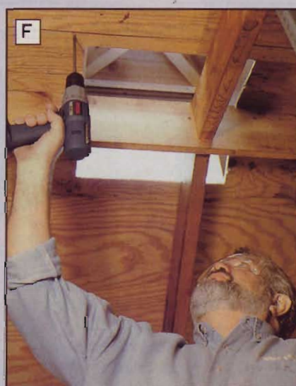
F Using a helper on the roof to hold the cupola in place, drive screws through the roof sheathing into the cupola corner posts.
