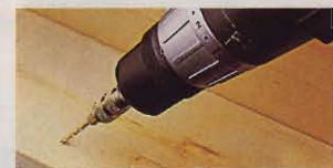
Drill pilot holes
