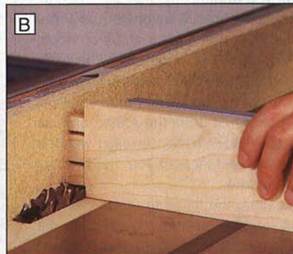
Switch to a dado blade to cut the tenons. Adjust the blade height as required.
