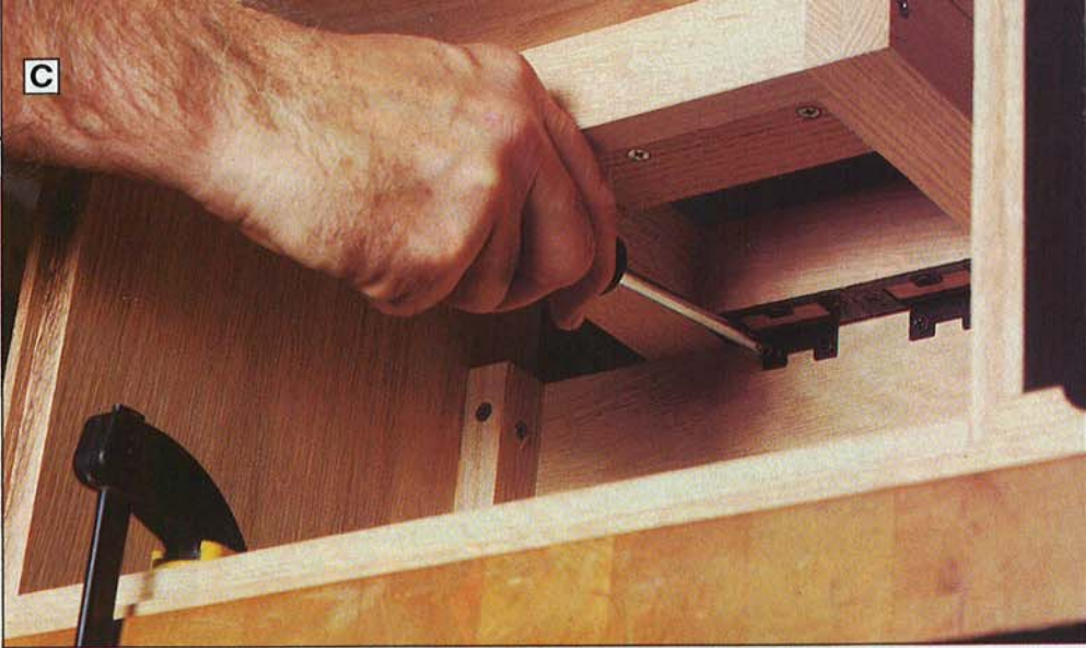
With the cabinet clamped to your workbench and working from the back of the cabinet, hinge the ironing board assembly to the inside spreader support (G).
