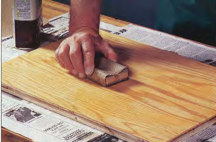
To create a slurry to fill the grain's pores, heavily coat the surface with a mix of natural oil and paint thinner, then vigorously sand with 100-grit paper.
