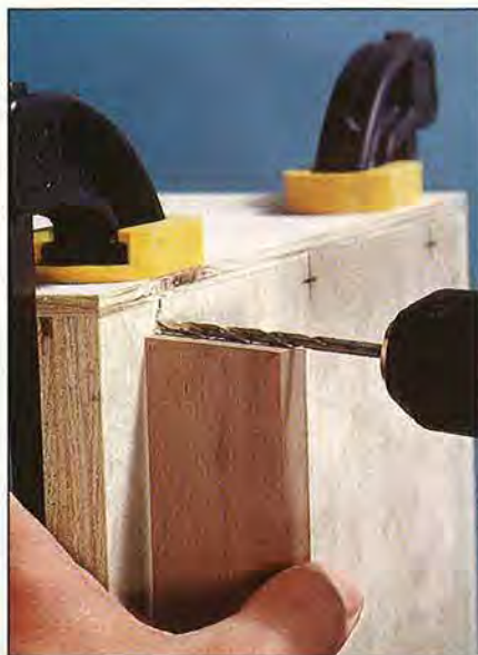
After marking the centerpoints 1\frac{1}{2} " in from the outside edge, use a 5^\circ drill guide to drill the angled holes.
