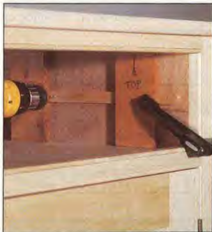
Use a pair of spacers to accurately position the guides. Then, drill mating holes in the kickers for attaching the guides.
