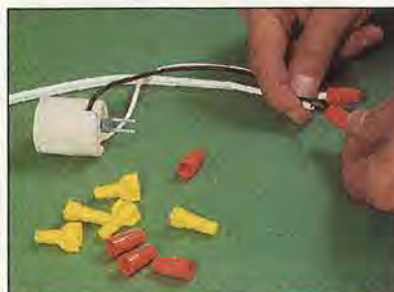
Twist conductors together before screwing on the wire connector.
