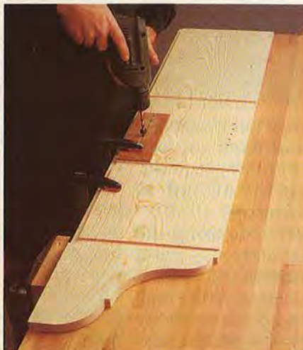
For equally spaced holes and level shelves, make a template and drill \frac{1}{4} " holes for the shelf pins.
