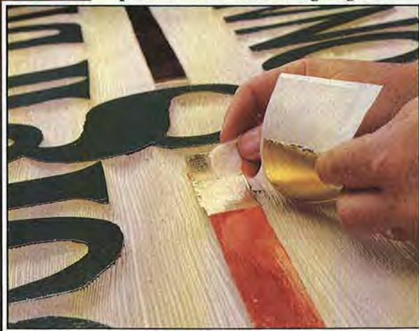
▲ Twenty-two-carat gold leaf adds to a sign's appeal and expense. Brent lays it down, then burnishes it in place.
