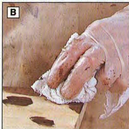
Apply a gel stain to areas prone to dirt and grime buildup.
