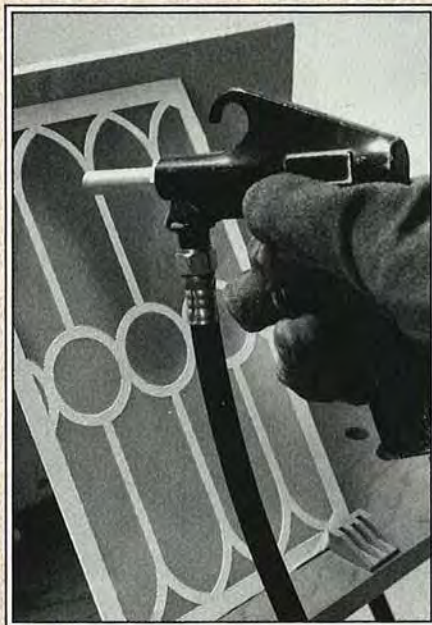
Sandblast the glass in overlapping sweeps for even coverage.
