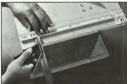
Position the drawer slide parallel to the bottom of the drawer.
