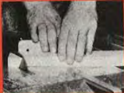
Making a compound miter cut.
