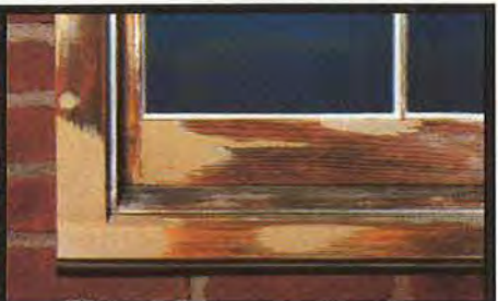
Rebuild rotted wood
