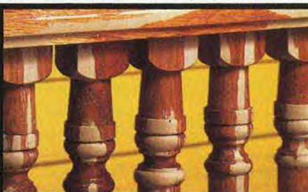
Restore damaged wood
