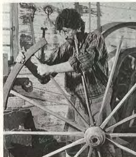
Colonial Williamsburg master wheelwright Daniel Stebbins fits a felly to a carriage wheel.
