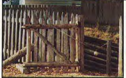
Pictured above, top to bottom: arbor gate decorating an alley entrance; Chinese fence corner gate; gate enhanced by massive posts; gate with mortised pales; decorative main gate; rough-hewn cedar paled gate showing common closing device with sliding iron ball.
