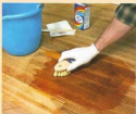
1] Mix the wood bleach (oxalic acid powder) with hot water, and scrub it onto the stain.
