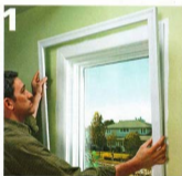
1] To install the frame, set it over the existing window trim, so the reveal is even all around. Check for gaps ( Fig. 2 ) before nailing the frame in place.
