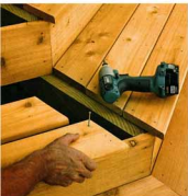
The treads are mitered at 22½° to wrap around the corner and secured with almost-invisible trimhead screws.
