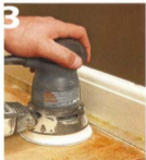
SAND THE EDGES Once the "field" is sanded, use a random-orbit sander to sand the edges of the floor.
