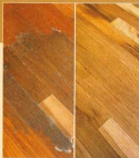
After scrubbing this water stain with a wood bleach solution and letting it dry overnight, it cleaned right up.
