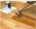
3] To make sure acid residue won't react with the finish, brush on a thin test coat of finish.
