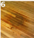
6 REMOVE STUBBORN STAINS If any stains remain after sanding, use wood bleach to remove them (see page 63).
