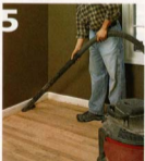
5 VACUUM DUST Once the entire floor is sanded, vacuum the dust using a
