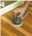
SAND LIGHT & QUICK Sanding between coats removes any dust. Use 240-grit discs on a random-orbit sander.
