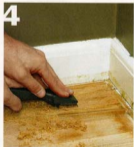
4 SCRAPE THE CORNERS Use a paint scraper to remove finish in the corners and other areas the sander can't reach.
