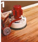
SAND THE "FIELD" After installing 36-grit discs on the sander, sand slowly back and forth to remove the finish.
