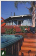
A The elevation of the deck is used to integrate a spa without the need for additional structure.
