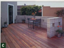
C Even a large, unbroken field of deck boards seems inviting thanks to the rich color of redwood. Here the homeowner made use of cinder and glass blocks to define an outdoor dining area. The door in this photo leads directly to the indoor cooking and dining space.
