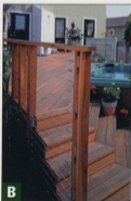
B Cables strung between redwood posts and secured with turnbuckles create a striking border to the deck.
