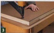
▲ Once all of the inner core pieces are fastened, glue the second skin on top of the panel. Here again, align the edges of the skin flush with the core pieces and tack it in place.
