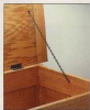
▲ The hinges for the lid are "aged" to look like antique bronze (page 62). A chain prevents the lid from being opened too far.
