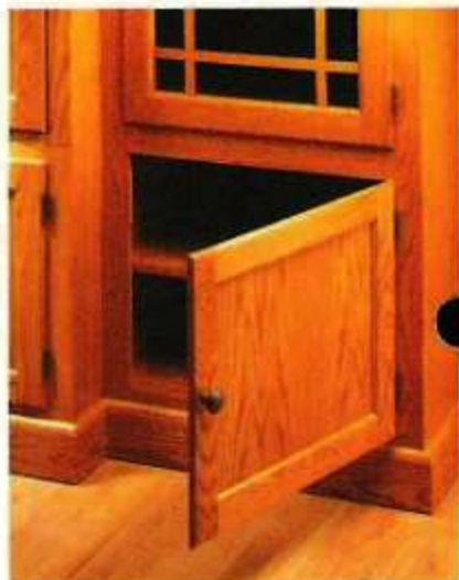
▲ The lower frame and panel inset door for the side cabinets are identical to the lower doors of the TV cabinet.
