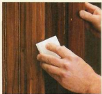
A Little Wax. Next, a block of paraffin wax will help expose the layers later on. Just rub areas that would normally be worn and the paint to follow will sand off easily.
