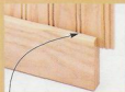
▲ When the beading detail drops behind the rails, it creates dark shadows and a "fuzzy" joint.
