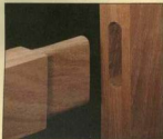
Frame. While many doors use joinery that must be reinforced with dowels, the frame on this door is joined with simple but strong mortise and tenon.
