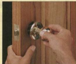
Installation. The last step to installation is the easiest — adding the handle and dead bolt. But before this can happen, the door has to be trimmed to size and hung in place.
