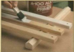
Oil-based Primer. Before screwing the seat slats to the Bench, they are first primed with an oil-based or alkyd primer.
