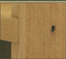
Square-cut nails are an authentic detail. They go into pre-drilled holes, then are "set" with punch before sanding.
