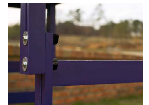
The 1/4-inch slot in each leg piece allows the height of the table to be adjusted.
