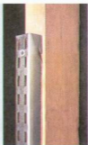
▲ Screw Mount. You can mount the uprights directly to studs or block walls using screws.
