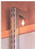
▲ Hook. If your ceiling is unfinished, you can hang the uprights from the top plate using the hooks.
