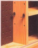
▲ Shelf Pins. Removable shelf pins are used to support the adjustable shelves inside the pegboard storage cabinet.
