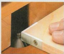
the holes for the screws. Here again, a support block prevents the soft metal from "breaking" out the back side of the angle. Once the angle is installed, the edge can be shaped by routing with a carbide-tipped router bit.
