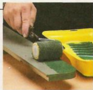
Step 2. After covering the edges, roll the paint on the faces, making sure to lay down a good, "wet" coat.
